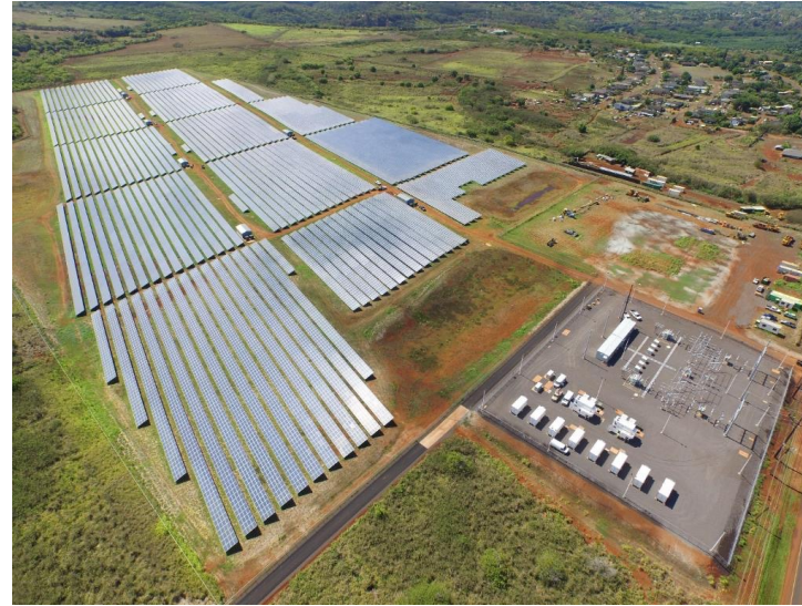
Saft 6 MW / 4.2 MWh ESS Kauai - Grid Stability
